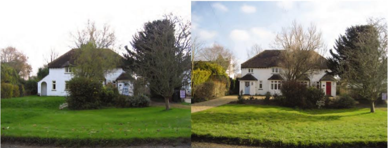
Sensitive joint scheme design in Itchenor for the extension of a pair of semi-detached houses; before and after
